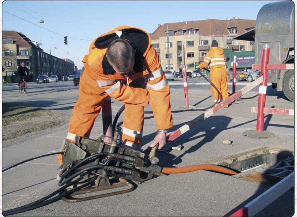
John Hansen and Søren Dam from Petri & Haugsted A/S prepares to flush a new cable into an existing pipe in central Copenhagen. John Hansen connect the water supply hose while Søren Dam connect it to the water tanker.
